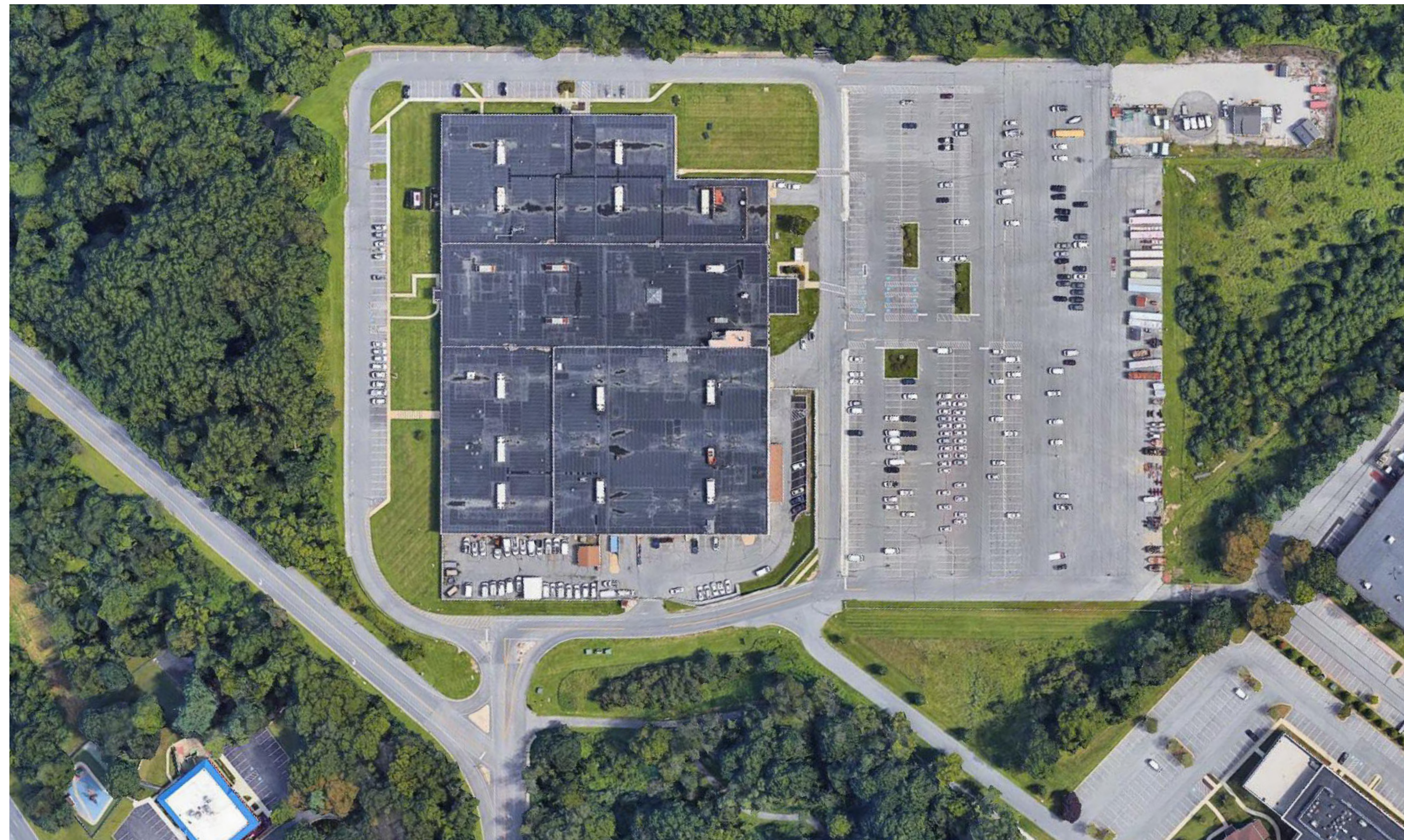
EXISTING SITE CONDITION
